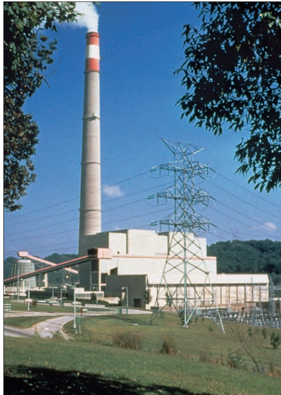
Bull Run thermoelectric power plant, Anderson County, Tennessee. (Photo courtesy of Tennessee Valley Authority.)
