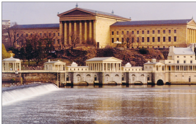
Fairmont Water Works (1815–1911), Philadelphia, Pa. (Photo courtesy of Philadelphia Water Department.)
